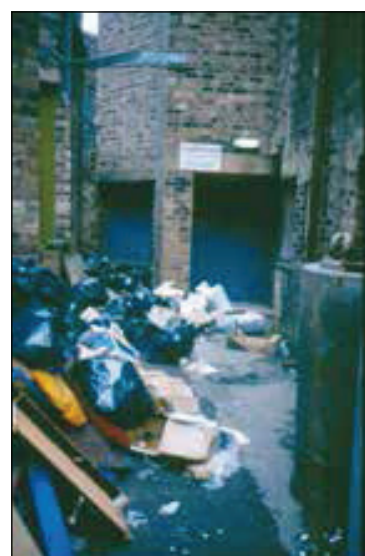
Figure 9: A blocked escape route
